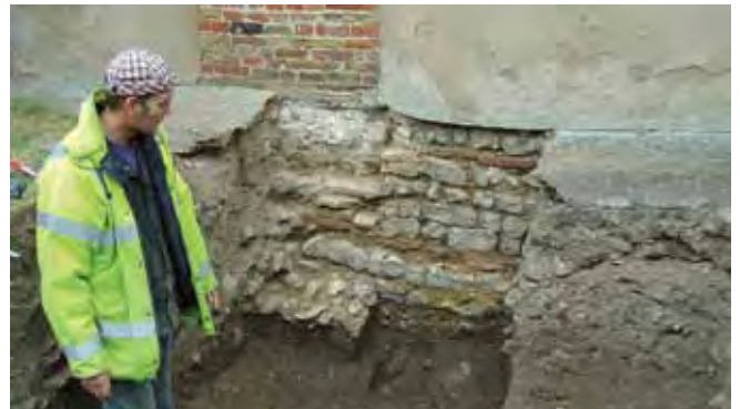
Excavation of the trench against the south wall of Caistor church in progress showing facing flints in the wall which look Roman.
