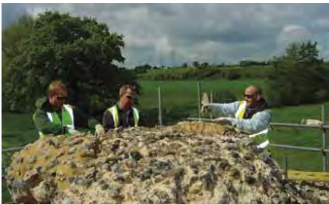
Adrian Fox and some of the team from W.S. Lusher & Son rough racking the top of the Roman western bastion at Caistor.
