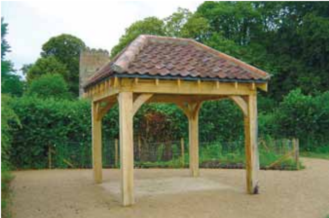
One of the two new timber-framed shelters designed to hold the interpretation panels to be installed for a spring opening at Burgh Castle.
