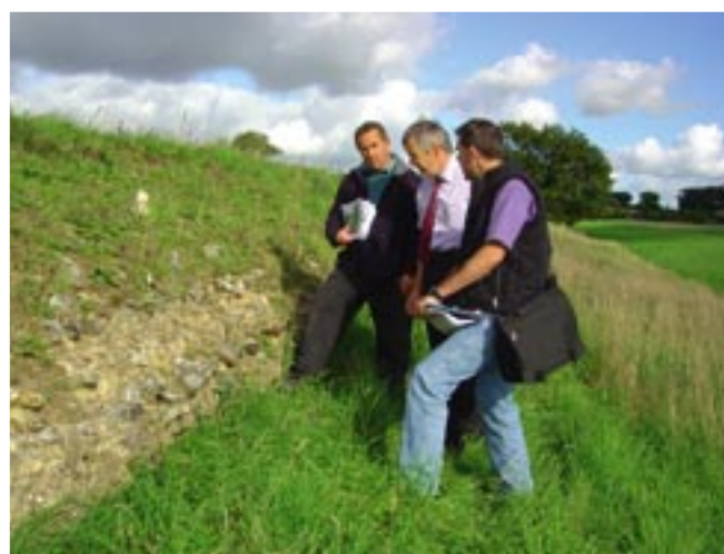
A site meeting at Caistor between David Watt (right), the Trust's building surveyor, Mark Lusher of W.S. Lusher & Son and his site foreman Adrian Fox (left) at the south wall discussing how best to carry out the necessary repairs to the Roman stonework while at the same time causing minimal damage to the rare chalk-loving plants growing on the wall. Photo Peter Wade-Martins
