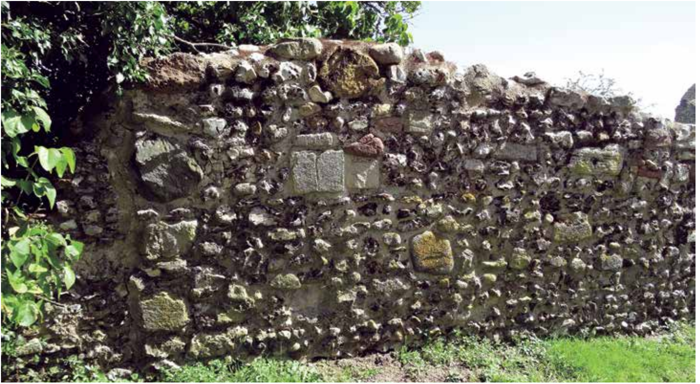
Image 12: The western boundary wall at Burnham Norton Friary
