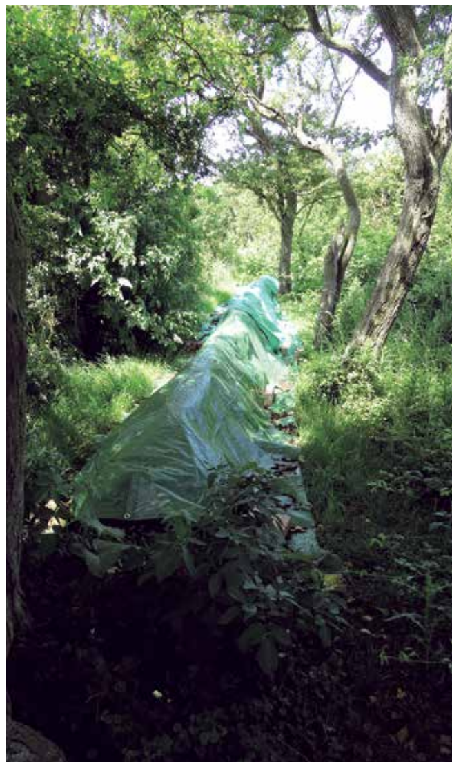
Image 10: St Benet's precinct wall during repairs showing overhanging shrubs.
