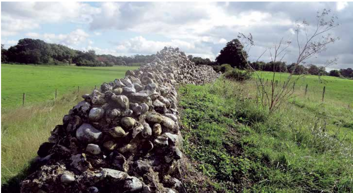
Image 6: Works to walls during 2015.
