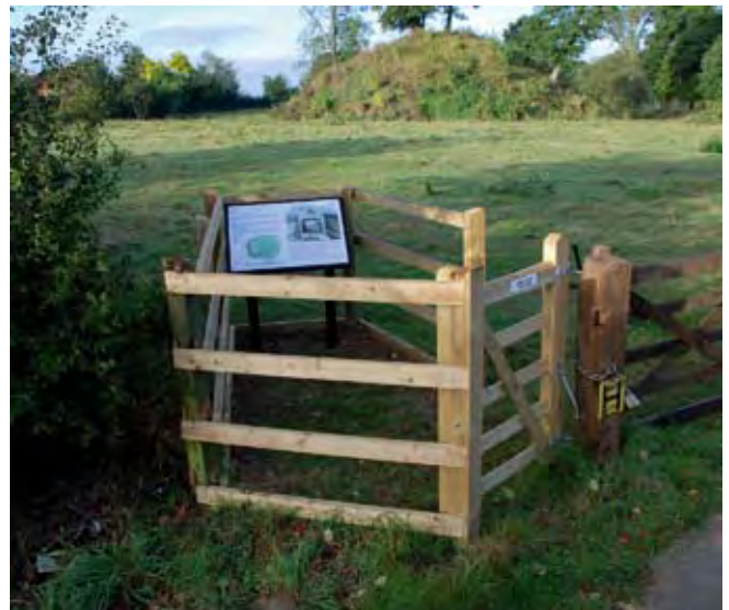
The kissing gate at Middleton with the new interpretation panel located within the frame of the kissing gate to prevent damage by cattle grazing on the castle mound.
