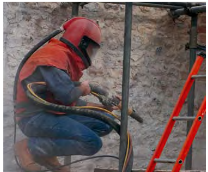
Sand-blasting the interior of the gatehouse to clean off modern whitewash.
