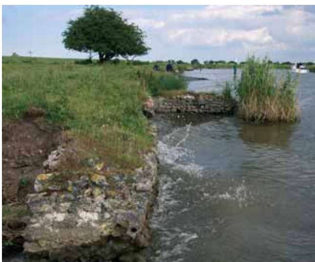
The wash from cruisers on the River Bure is doing considerable damage to the river bank at St Benets. Photo by Sue White
