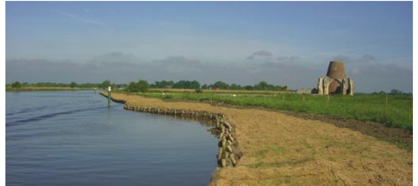
The fully-restored riverbank at St Benets Abbey. It is worth comparing this picture with the one on the cover of the 2004 annual report showing the site before work began. As the new ground settles it may be necessary to spread some more topsoil over the new matting, and it will then be re-seeded. Photo Peter Wade-Martins
