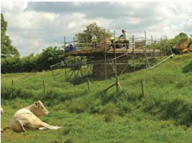
Conservation work begins on the Roman bastion overlooking the river at Caistor. A new flint and mortar cap is being placed over the Roman flintwork to protect the structure from frost damage.
