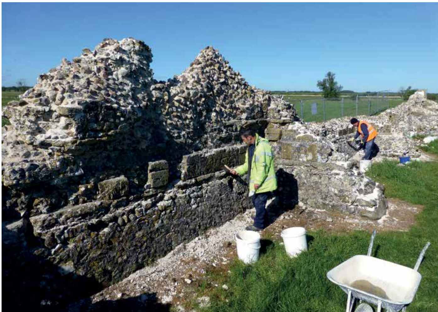
The conservation team repointing the panels of fine flint flushwork on the exterior face of the north wall of the church.
