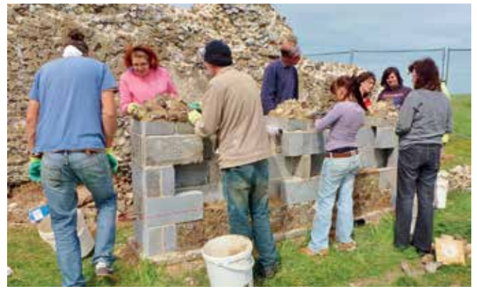
Participants on the workshop had a try at using flints to create panels of flint flushwork and rough racking on wall tops.
