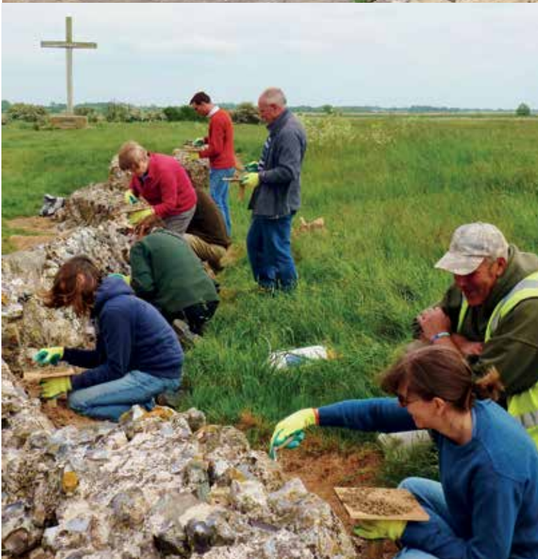
Re-pointing the south wall of the abbey church with Steve Martin, the R. & J. Hogg site foreman, maintaining a watchful eye on the work.
