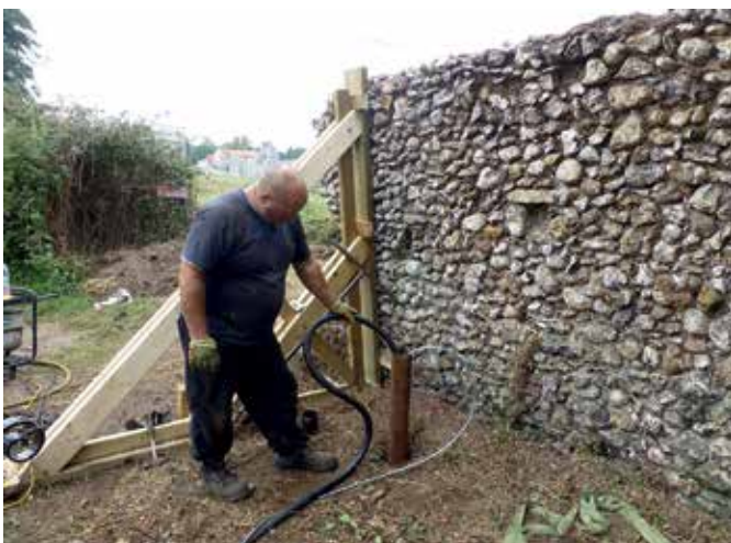
Piles are driven in with compressed air to support new buttresses on the river-side section of precinct wall.
