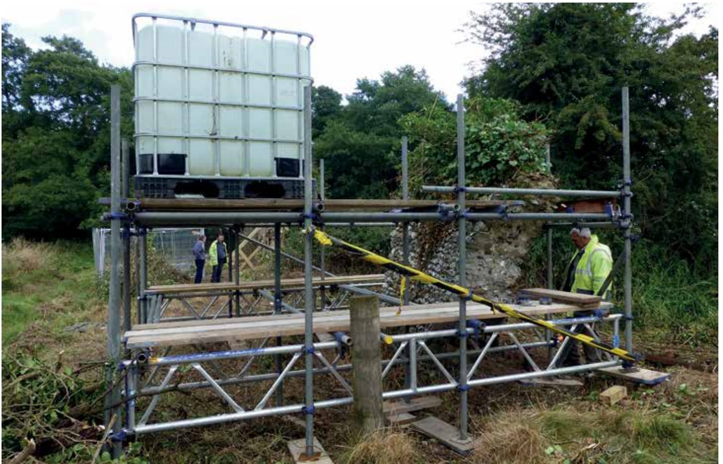
A clever system of water-filled weights has stabilised a leaning section of precinct wall while piles are driven in to support new buttresses.
