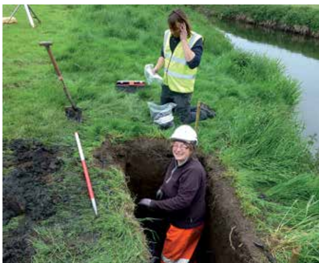
The construction of the footbridge involved cutting foundations down through the valley deposits into the underlying gravel. The trenches were dug by consultant archaeologist Heather Wallis who clearly enjoyed the experience! With her was Dave Bescoby who has made a special study of the alluvial deposits in the valley. He reports that from about 1.2 m down to 1.8 m there is a deep organic-rich layer of silts and peats representing a river edge marsh dating from the late Iron Age to c. 4th century AD.
