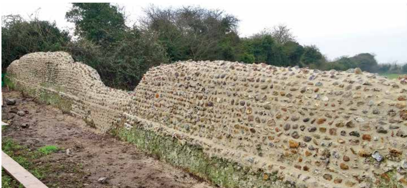
Fig 4: Burnham Norton, repaired section of east wall
